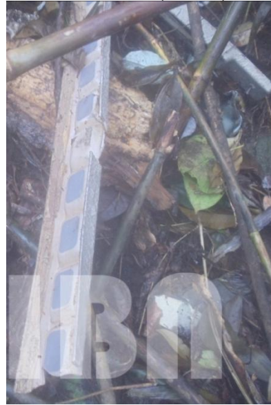
PANELS WITH FIRE DAMAGE
